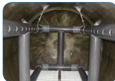
Looped lateral system - Inside view
