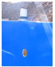
Use a 4" (102mm) hole saw and drill a hole for the pool light at a maximum depth of 400mm below the top of the finished deck level.
