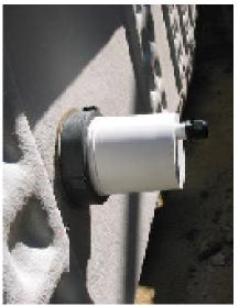
Firstly ensure that there is a flat surface at the rear of the fibreglass shell so that the lock ring will tighten up properly with the use of a strap wrench (available through Aqua-Quip).
